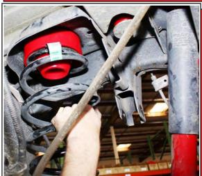
Install the coil springs on their designated sides of the vehicle. A spring compressor may be needed to ease the installation of the spring. Lower the vehicle to ride height. Reconnect the endlinks and lower shock mounts and torque bolts to factory specs. It is recommended to have your vehicle aligned after the installation of these parts.
